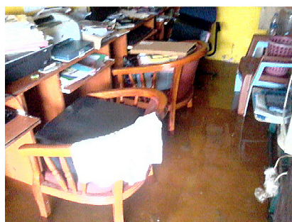
Computer and furniture washed out
